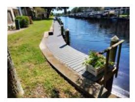
Note: This Reserve Item was refurbished in 2020 with new joists and decking, the pilings were reinforced. It is estimated that this will extend the life of the current structure until the seawall behind it is reconstructed.
